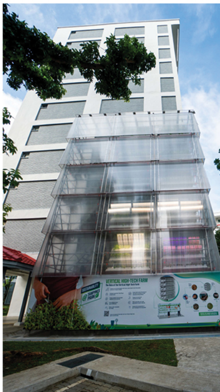
Vertical High-tech Farm – Housing Development Board – (Public Housing), Singapore
